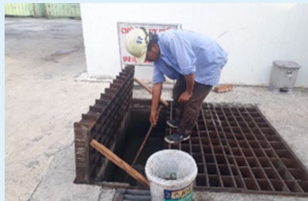
Cleaning, dredging ditches, manholes
