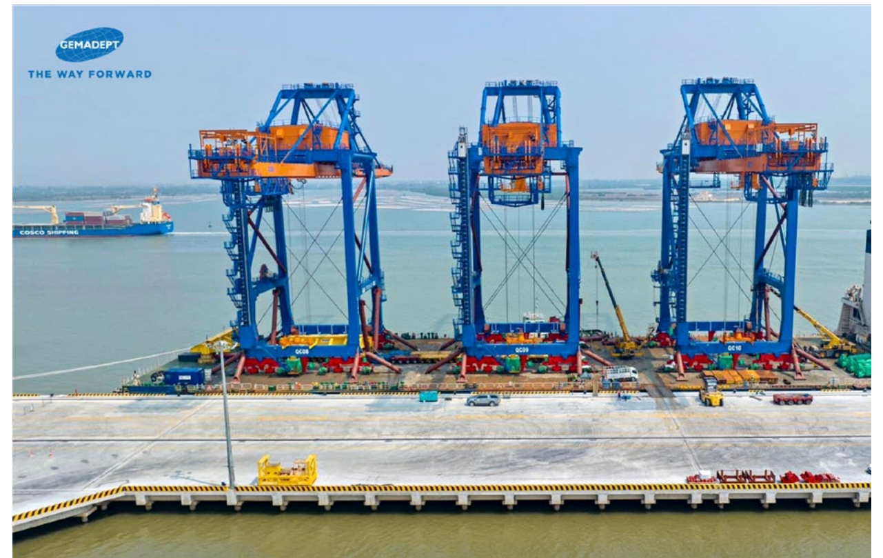
Electric-powered STS cranes are being installed at Phase 2 of Nam Dinh Vu port.
