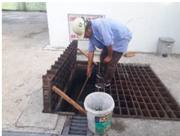
Cleaning, dredging, utilizing access holes to collect water
